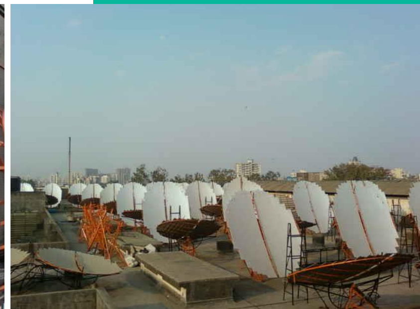
Scheffler solar thermal concentrators
