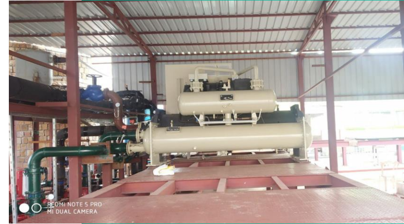
Vapor compression screw chillers with VFD
