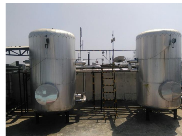
Associated storage tanks for hot and chilled water
